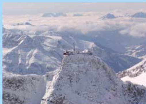
The Sonnblick observatory in its present form. Energy supply is electrical, the tower in the middle serves as wind mast and exhaust point for inhouse emissions.
