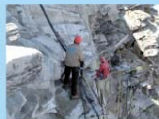
Temperature changes in the rock caused permafrost to recede. The stability of the summit was endangered. 105 stainless steel anchors were placed underneath the observatory.
