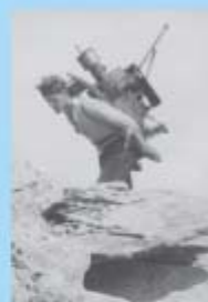
Carrying material for the cable car in 1956.
