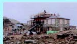
The Institute "Angelo Mosso" during the reconstruction after the fire on June 2000.
