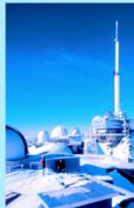
A view of the Observatory
